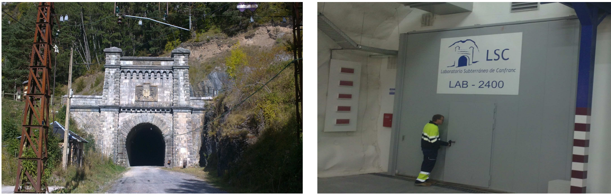
Fig. 4.3: Left, secondary or auxiliary entrance to the tunnel. Right, main entrance to the LSC and one of the researchers.
