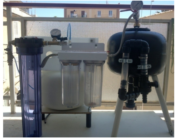
Fig. 6. The anaerobic digester system.
