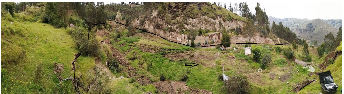
Figure 12. A panoramic lateral view of the Pujilí landslide taken from the right flank shows the scarp failure at the center of the picture (movement from left to right, arrow). In the bottom-right corner of the picture, the HVSR geophysical equipment is placed for survey.
