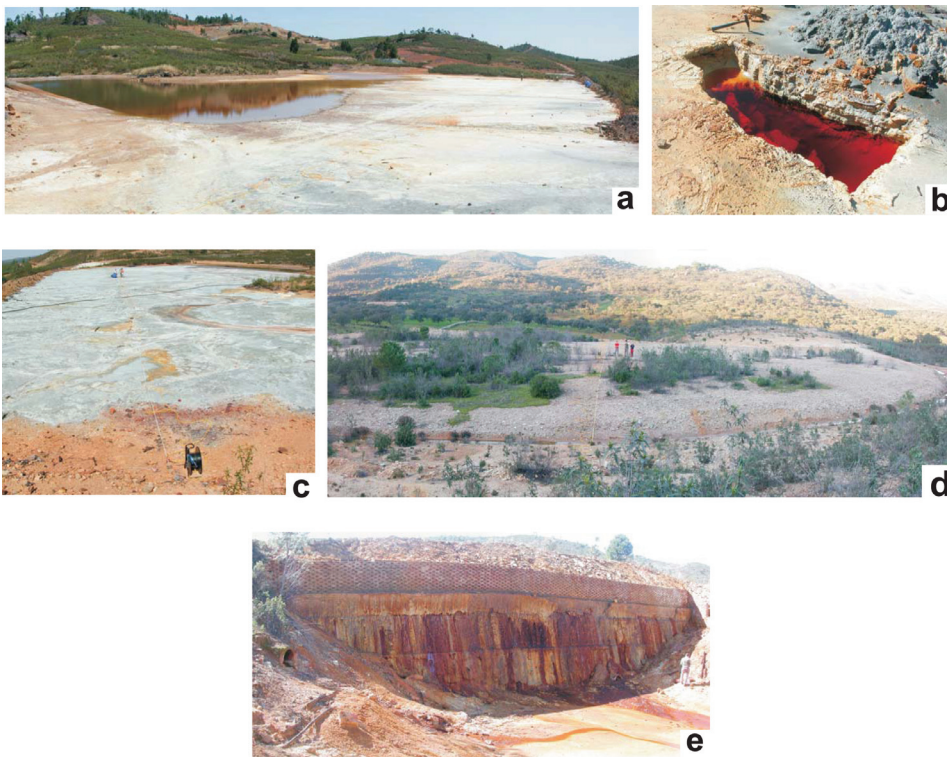
FIGURE 2 a) General view of the Monte Romero abandoned mine pond; b) small ditch showing the water level. Note the colour of the acid water caused by the iron content; c) electric longitudinal profile at the easternmost mine pond (profile 3); d) main view of the Mina Concepción abandoned mine pond; e) detail of the containment dam with acid water drainage.
