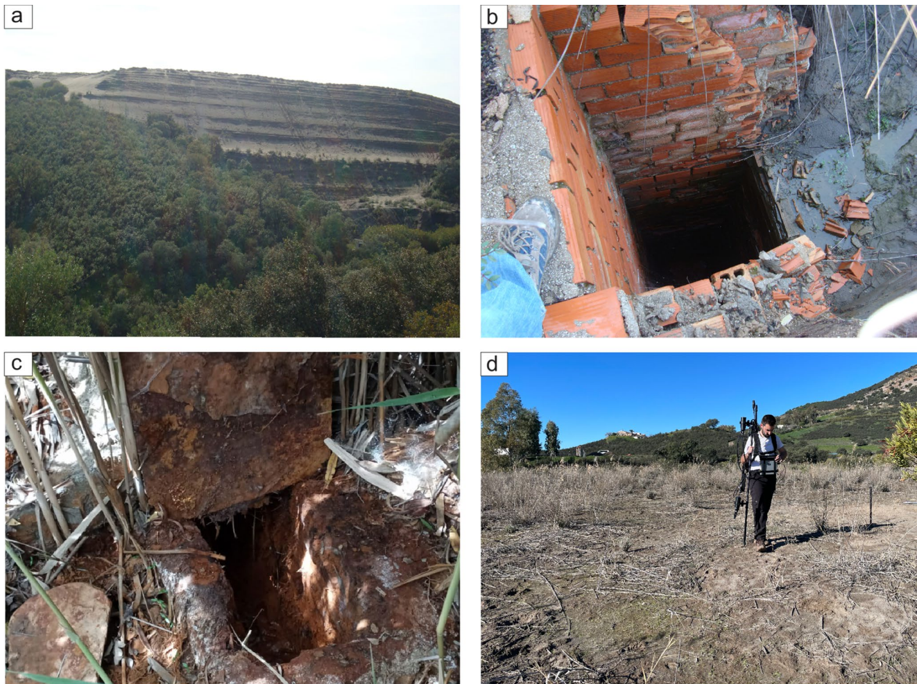
Fig. 3 Photographs. (a) General view of the tailings dam. (b) Upper part of the chimney drain installed in the tailings dam. (c) Details of the drainage at the foot of the tailings dam. (d) Field procedure used for magnetic data collection using the GSMP magnetometer
