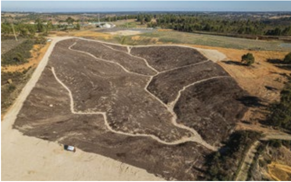
Figure 3. New geomorphic design of the intervention area, already with its two-layer soil cover, combined with three open limestone channels that direct flow through the area.
