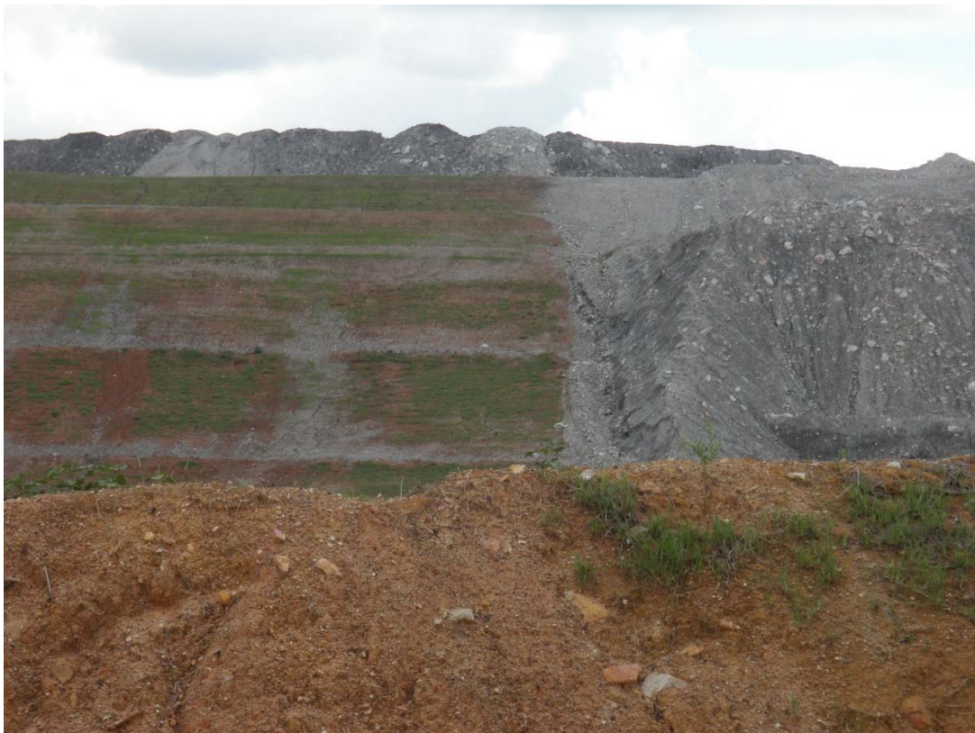
Figure 7. A reconstructed landscape with benches and contour banks and initial revegetation. Rills and gullies can be observed (top). A partially rehabilitated hillslope with benches and contour banks displaying the underlying material and initial dump shape (bottom).
