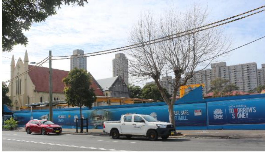
Figure 1.8: Construction Site of Waterloo Metro Station 2021 (Source: Dore 2019).
