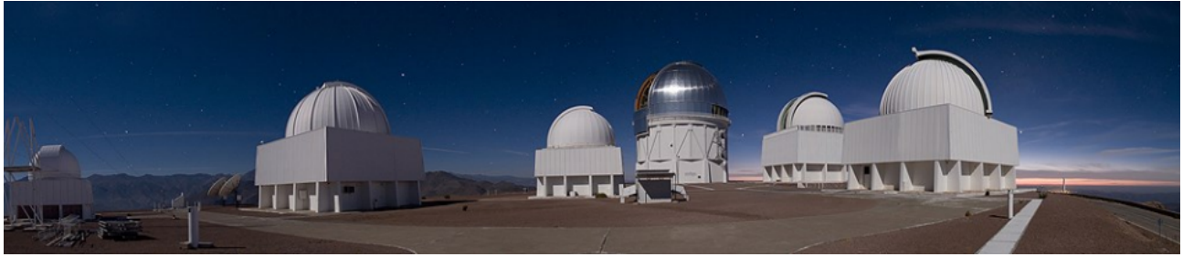
Figure 4.3: Cerro Tololo Inter-American Observatory. Picture Credit: Dark Energy Survey Collaboration.
