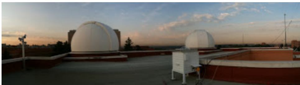
FIGURE 2.1: AstMon UCM as installed in the roof of the physics building at Universidad Complutense de Madrid, Ciudad Universitaria.
