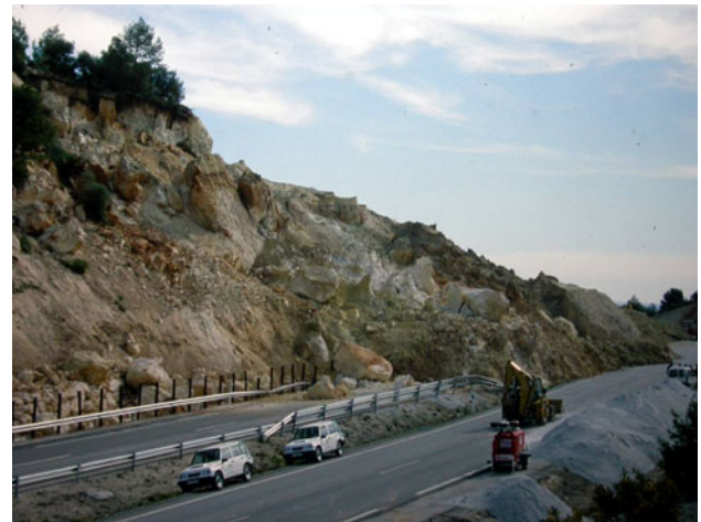
Fig. 3 Panoramic view of the toe of the Diezma landslide during the 2001 collapse over the A-92 motorway, which was closed for several days
