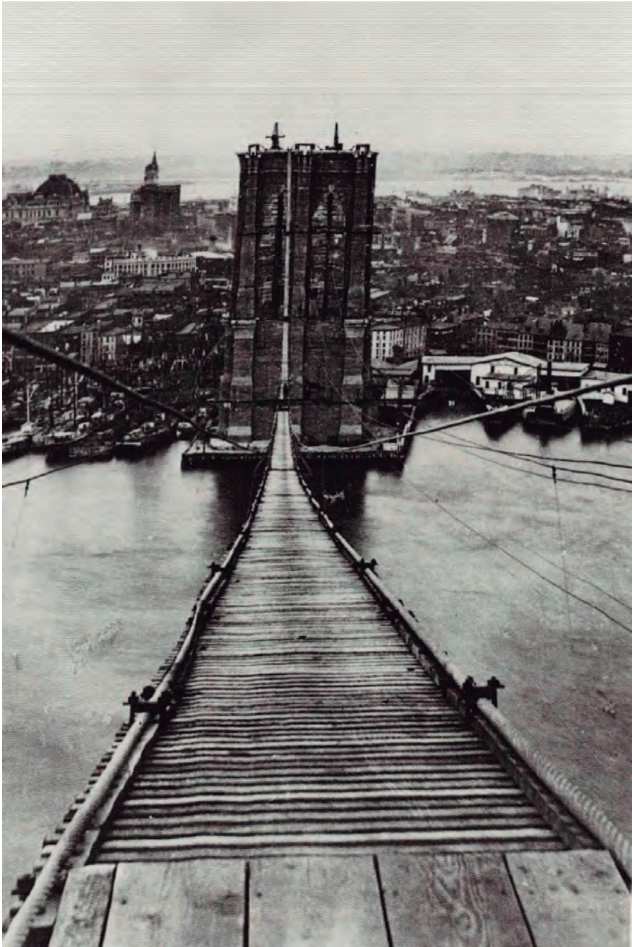
Anónimo, Brookling Bridge under construction , ca. 1869. Nueva York, Public Library.
