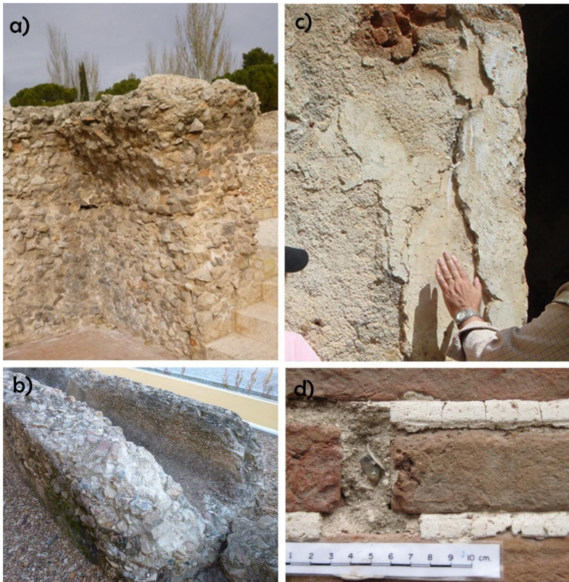
55 Figure 1. Examples of aerial lime mortars/plasters in ancient and historic buildings in Spain. a) Wall 56 built with mortar and limestone pebbles (> 10 cm size) in the Roman city of Complutum, Madrid; b) 57 Part of a channel from the San Lázaro Roman aqueduct, Mérida; the base was built with aerial mortar 58 and limestone pebbles, with several layers of aerial and hydraulic rendering mortars; c) Various layers 59 of rendering mortars applied on a wall in the Monastery of Santa María la Real in Pelayos de la Presa, 60 61 62 63 64 65
