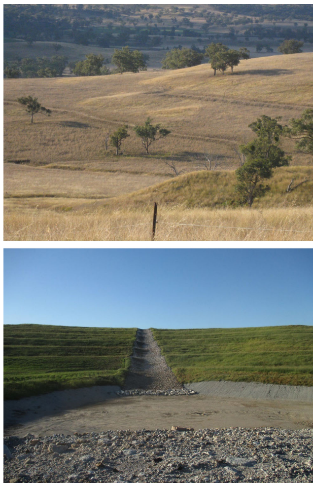
FIGURE 1 An agricultural landscape with contour drains constructed in 1980 with little erosion and receiving some maintenance and repair after a major storm event (top). A post-mining landscape constructed in a series of hillslopes (lifts) with contour drains directing runoff to a rock-lined channel (bottom). All sediment is contained within a sediment pond at the base of the slope. This landscape is hydrologically and sedimentologically disconnected from the surrounding unmined landscape.
