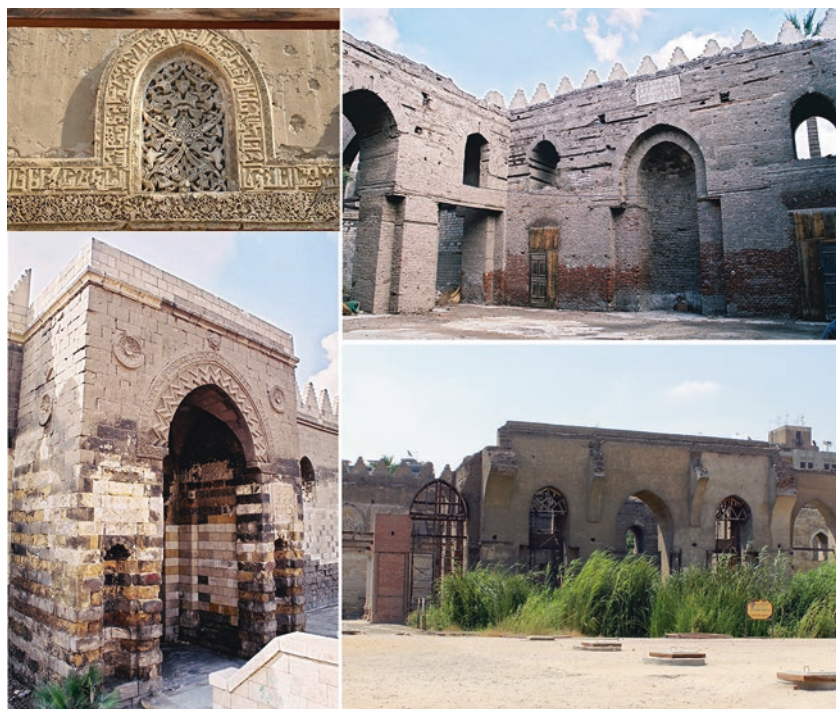
Fig. 3.2 Mosque of Sultan al-Zāhir Baybars, Cairo, in its state in 2019. (a) Epigraphic decoration and window. (b) Interior of the maqṣūra . (c) North-eastern gateway. (d) North face of the maqṣūra with the springing of four arches of the triple aisle basilica leading to the courtyard (Photos by the author)
