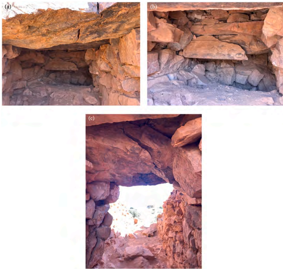
Fig. 6. Different fracture modes observed in the monumental complex: (a) detail showing an interior lintel fractured in mode I at the entrance to a chamber; (b) detail of a mixed-mode open fracture inside one of the chambers; (c) detail of a mixed-mode open fracture on one of the corridor lintels.
