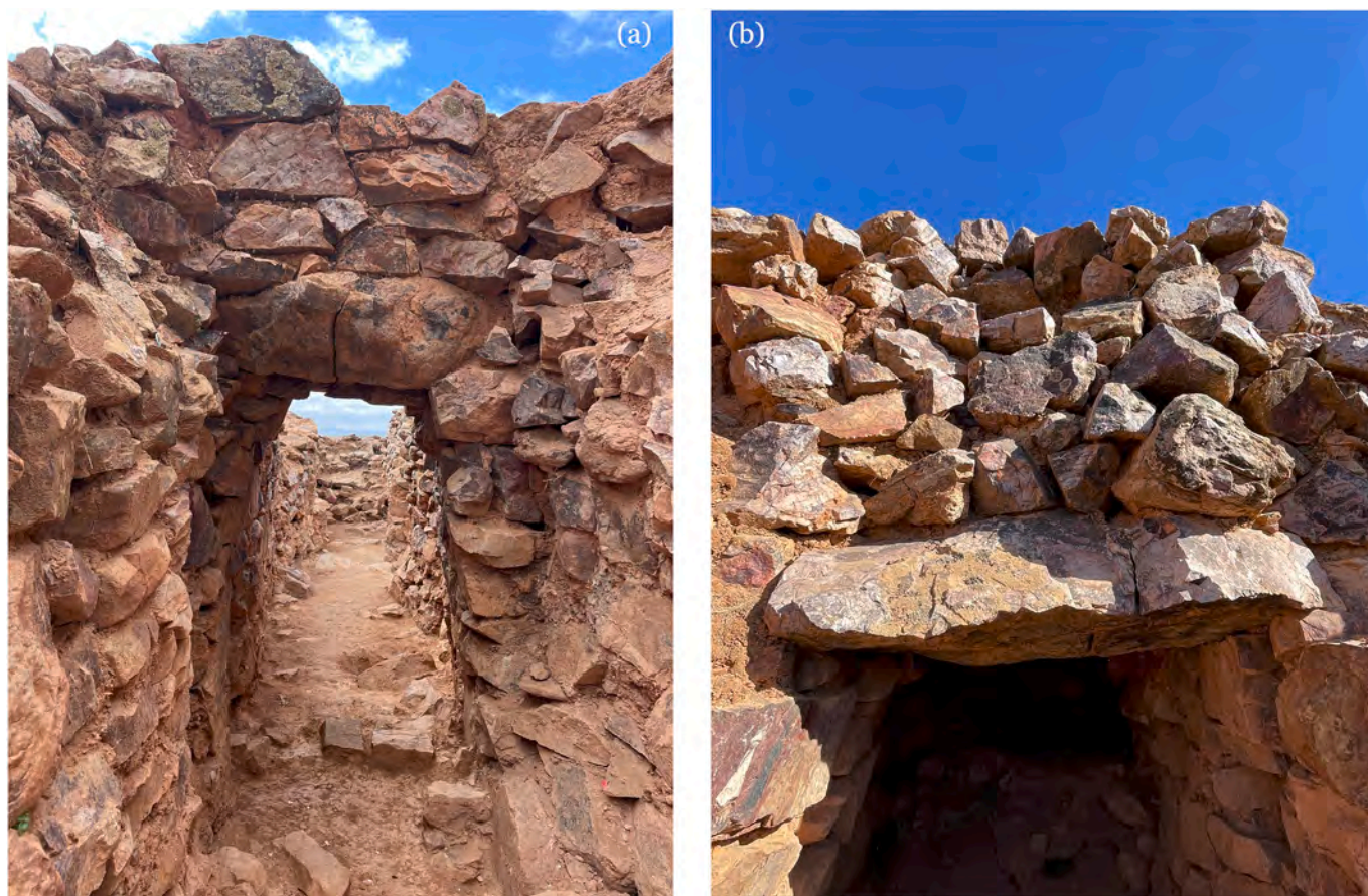
Fig. 5. Monumental spatial design: (a) large lintel with oversized cross-sections in a corridor; (b) large lintel with oversized cross-sections and heavy covering at the entrance of a chamber.
