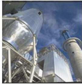
Photograph: TIRME, domestic waste incinerator at Son Reus, Majorca.
