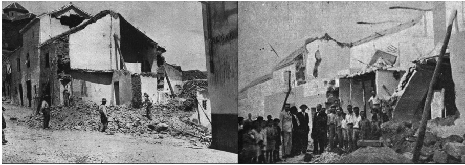
Fig. 22 Example of building collapses near the Castle Hill after the 1930 Montilla earthquake
