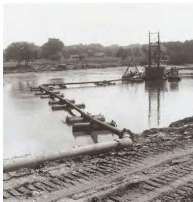
Figura 2. Monument with Pontoons: The Pumping Derrick. Robert Smithson (1967)
